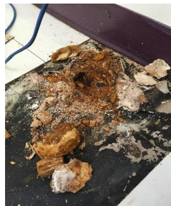
Image 1.2 Water damage under lower-level tiles
